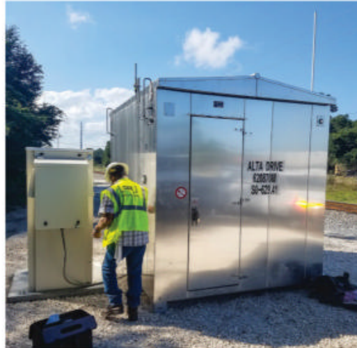
ALTERGY'S HYDROGEN FUEL CELL SYSTEM PROVIDES CLEAN, QUIET BACKUP POWER TO RAILROAD SIGNALING, SWITCHING, AND GATE-CROSSING SITES.
